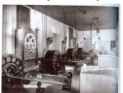
First 3-phase transmission system installed in Sweden between Hellsjön and Grängesberg 1893 voltage 9650 V, 70 Hz, 70 kW
